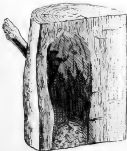
Fig. 325.—Trunk of an Oak ruined by the decay of the Stump of a Branch.
